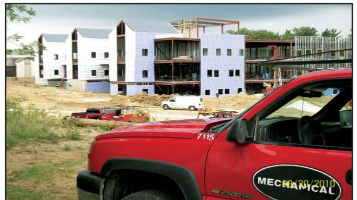
The building is currently under construction with all structural steel set in place with all floors poured. Exterior and interior wall framing is underway along with the rough in stage of all mechanical and plumbing systems. Fabrication of several pump skids have recently been completed and have been delivered to the site and the remainder of the mechanical room fabrication is underway as well.
