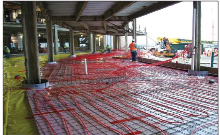
**Above: Pex tubing for in-floor radiant heat at the Silver Cross Hospital Entry.**
