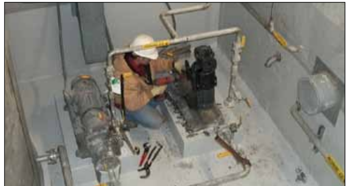
Tom France of Mechanical's Waukesha office meticulously inspecting work.
